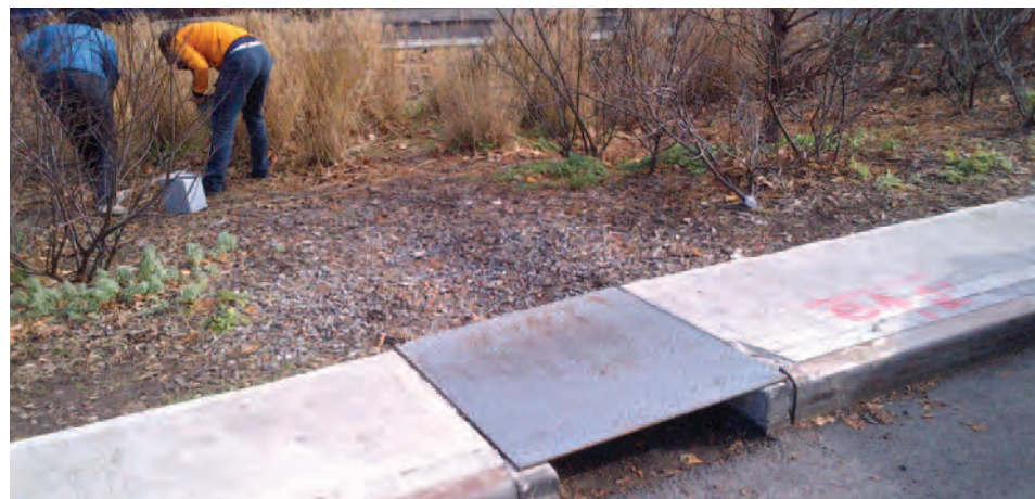
TOP: Enhanced tree pit in Brooklyn ABOVE: Enhanced tree pit in Philadelphia LEFT: Enhanced tree pit detail in the Bronx showing the stormwater inlet
