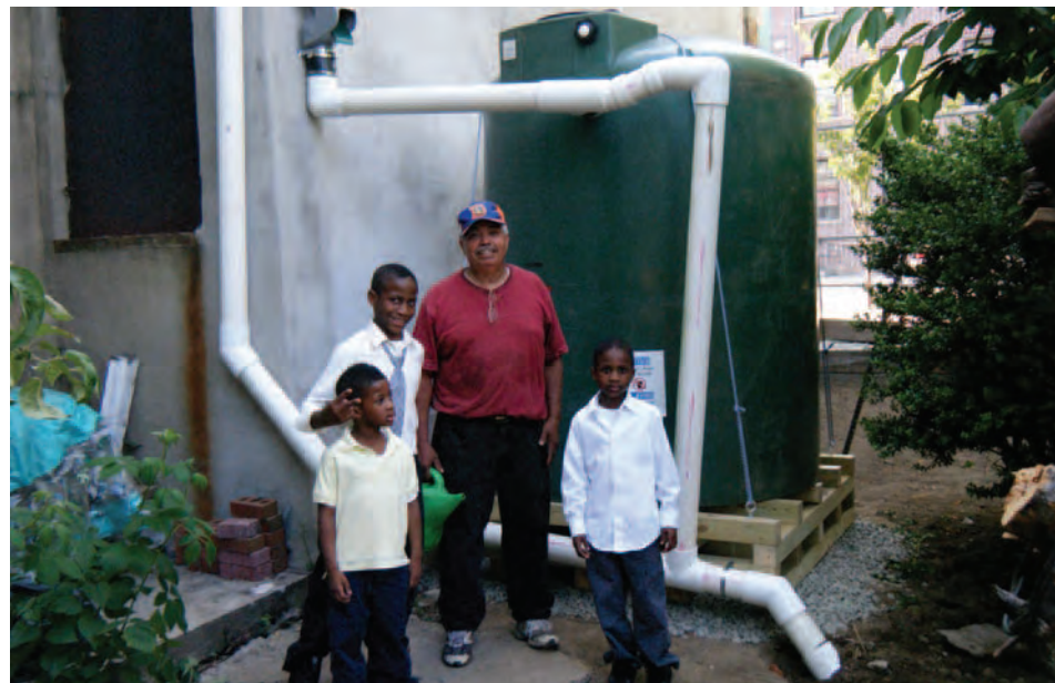
TOP: Rain water harvesting system in a Brooklyn community garden that captures water from both the adjacent building and the garden shade structure MIDDLE: Rain water harvesting system at a Staten Island residence LEFT: Rain water harvesting system in a Brooklyn community garden that collects rain water from an adjacent building
