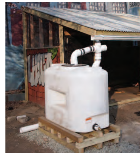
TOP: Rain water harvesting structure in a Bronx community garden ABOVE: Diagram of a typical rain water harvesting system LEFT: Rain water harvesting structure in a Manhattan school garden
