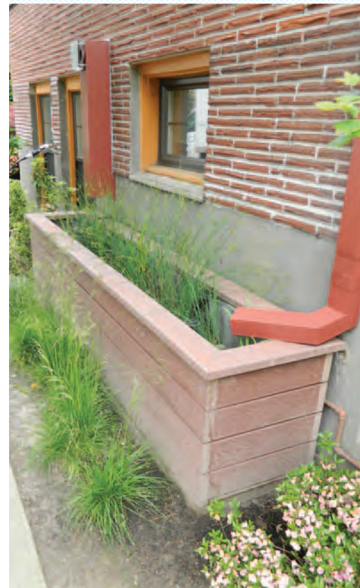
TOP: Rain Garden at the University of Minnesota-Duluth with native plants. BOTTOM: Downspout planter
