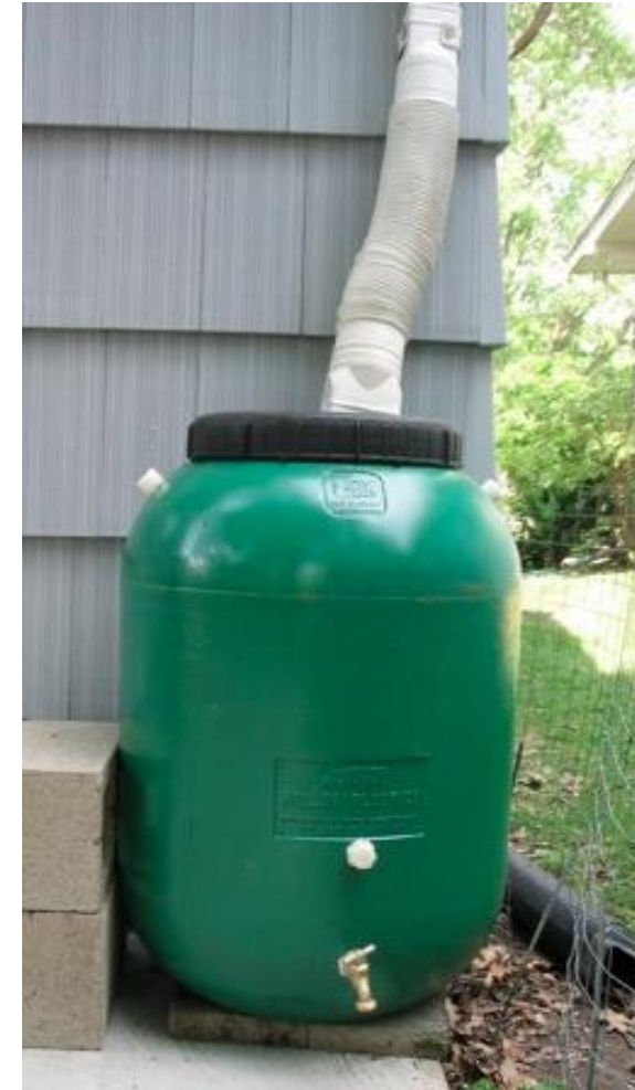
Rain barrels collect roof runoff for reuse
